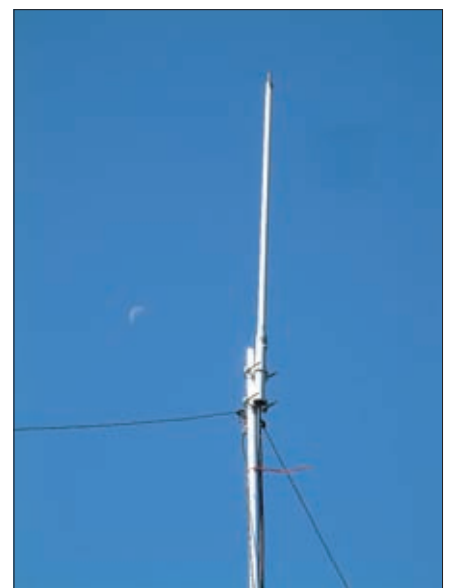
Fig. 2: A small triple-band (50/145/433MHz) antenna, which is ideal for local contacts. Notice how the support mast has also been used to support the feed-point of a wire antenna saving the visual impact of a second support.
