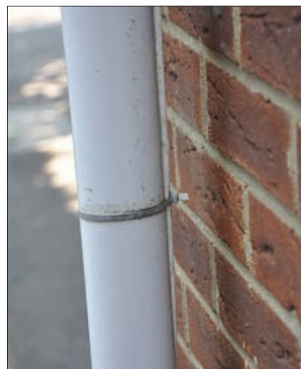
Fig. 6b: Using white feeder has helped hide the feeder still more – an even better idea would be to use matching cable ties!
