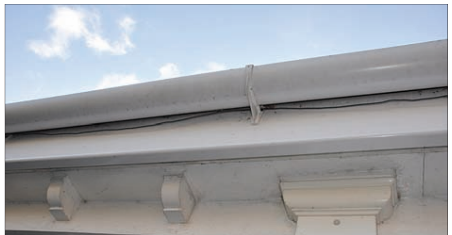
Fig. 5: A gutter mounted antenna. Changing the wire from black to white would make the antenna less visible, as would applying a little tension to prevent sagging.
